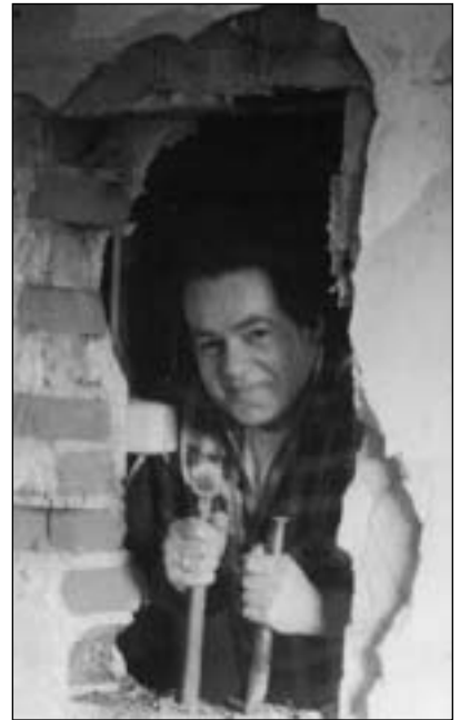
Working on the restoration of the Mizos' house in Höfen, Germany
